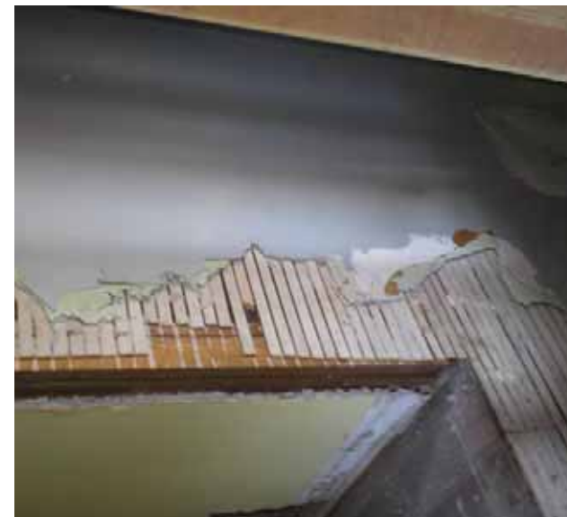
Asbestos was discovered during a 2011 home remodel in Portland. (Photo: Chris Zimmer)
